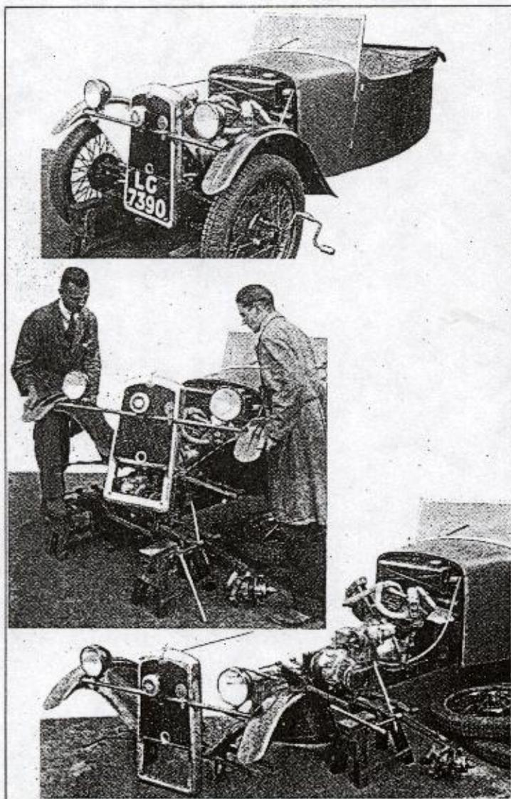
The accompanying illustrations show the simplest method of gaining access to the front portion of the Three Wheeler power unit.
